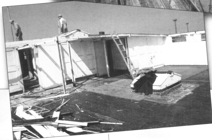
Left - Starting restoration work with the removal of non-original structures
